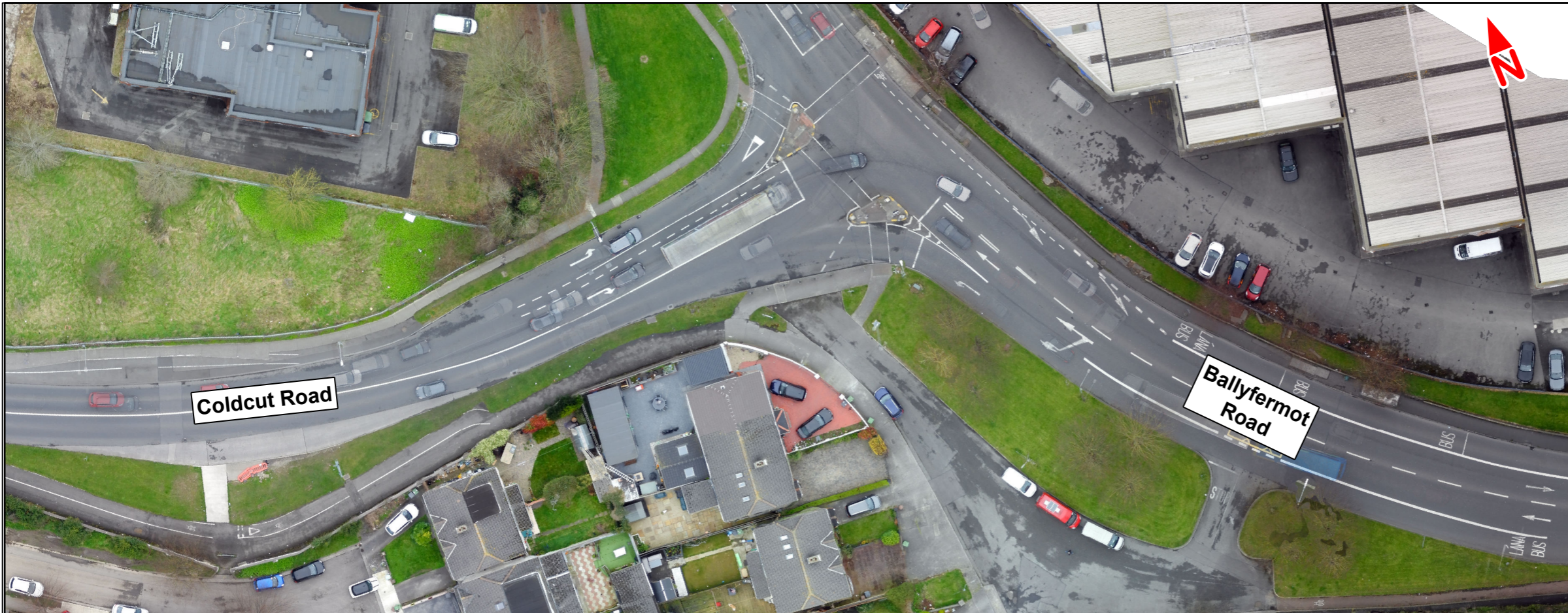
A) R833 Coldcut Road / R833 Ballyfermot Road Junction
