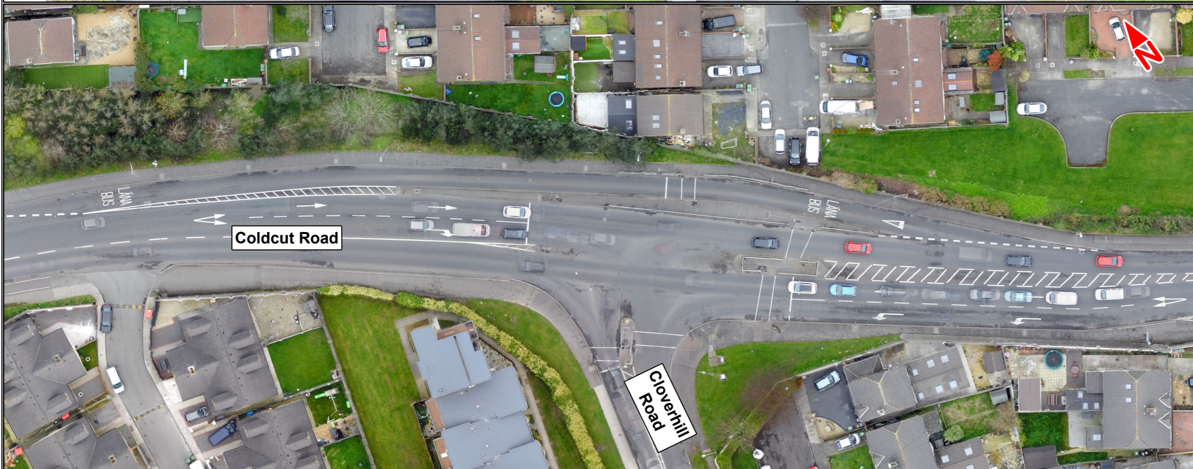
B) R833 Coldcut Road / Cloverhill Road Junction
